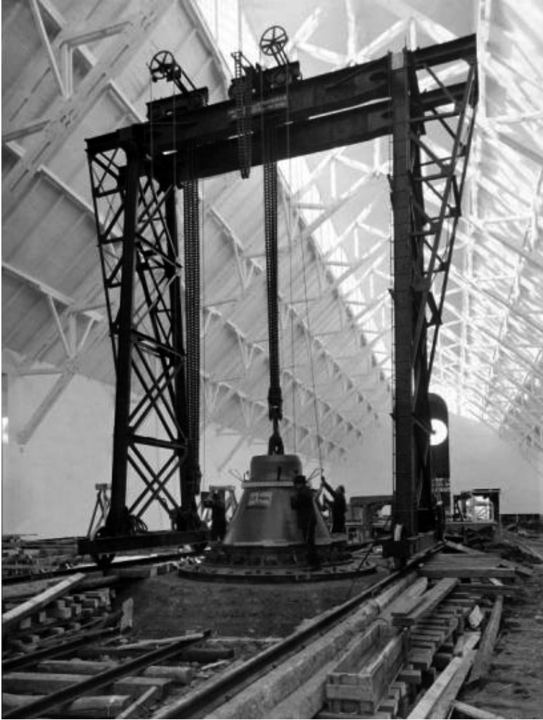
A cathedral of utility? The gun-carriage of a 135 ton coastal howit- zer gun being mounted in the middle of the Ma- chine Hall (GSM).
