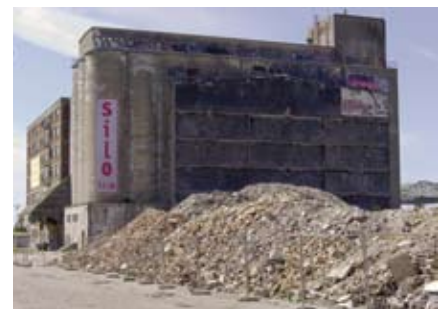
Silo 52, Islands Brygge
